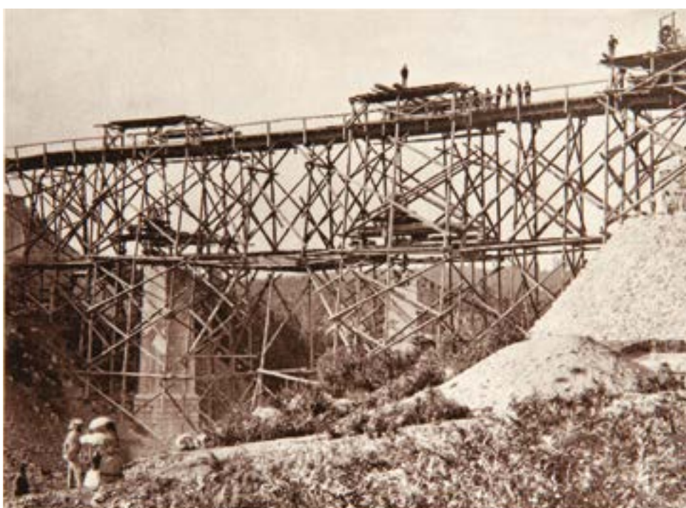
Construction of the railway viaduct near Globornica, 1872, M. Smokvina, Croatia in Historical Panoramic Photographs , Zagreb, 2001
