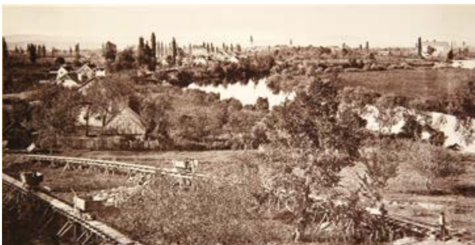
View of the Karlovac-Rijeka railway construction site, 1872, M. Smokvina, Croatia in Historical Panoramic Photographs , Zagreb, 2001
