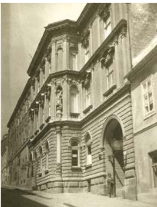
First Croatian Savings Bank building, 1642, MGZ
